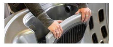
**Step 3:** Remove the pleated cartridge(s) by turning the filter core cap(s) counter clockwise then sliding the cartridge(s) upward from the filter core.
