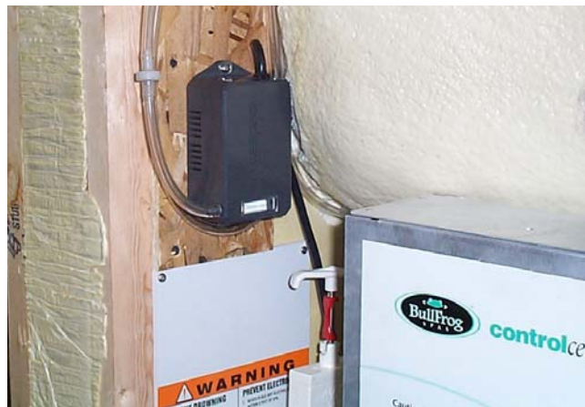
(Figure Y) Ozone Sterilizer Location
